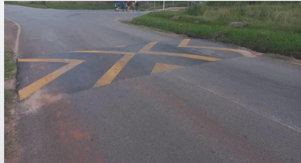
Installation of traffic calming speed humps
