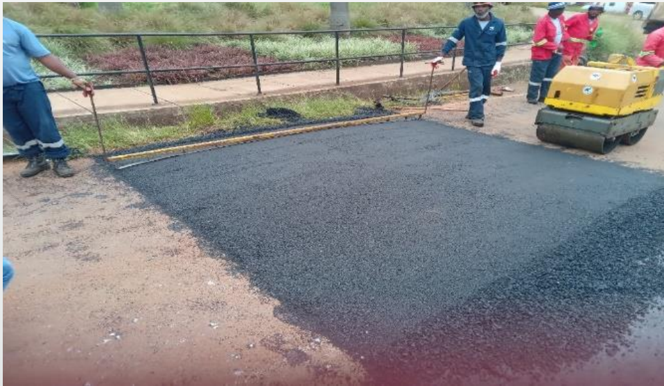
Installation of traffic calming speed humps
