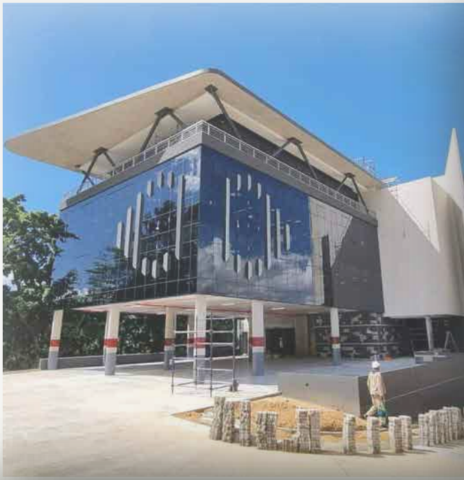
Figure 3 Progress at FNB head office site
