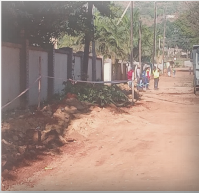
Figure 4: Clearing and grubbing of Lonyoni Road.
