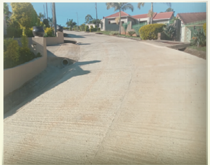
Figure 7: Complete Road at Umdoni Township
