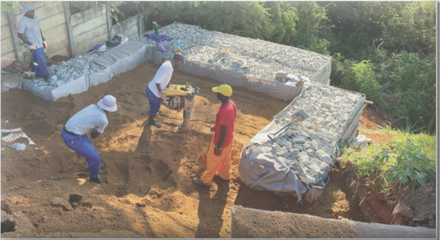
Figure 8: Construction of Gabions at Umdoni Township.
