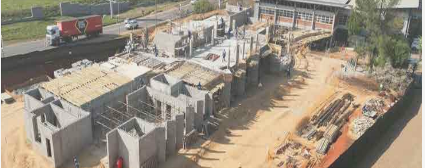
Figure 1: Progress at EWSC office extension.
