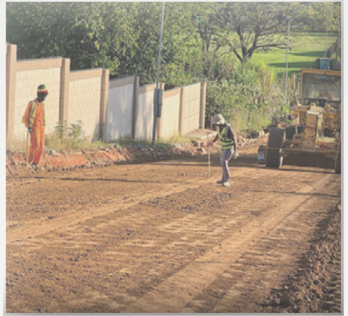
Figure 6: Progress of the rehabilitation of Mpumalanga Crescent Road in March 2023
