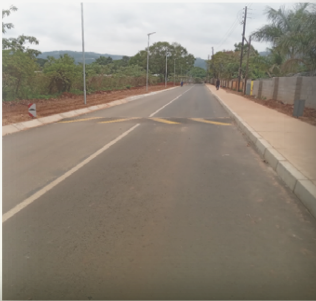
Figure 5: Completed Lonyoni Road.
