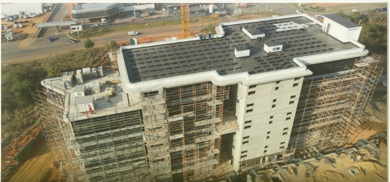
Figure 2 Progress at the ESCCOM site
