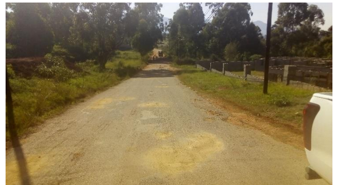
Figure 22: Potholes on old road
