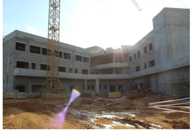
Figure 15: Complete blockwork
