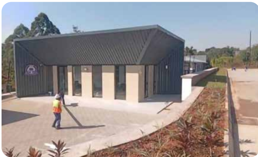
Figure 9: The completed Lubane Savings and Credit Co-operative Society office in Ezulwini.
