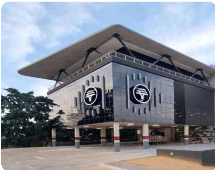
Figure 10: The completed FNB office in Ezulwini.
