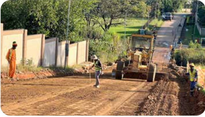
Figure 4: Processing of pavement layers.
