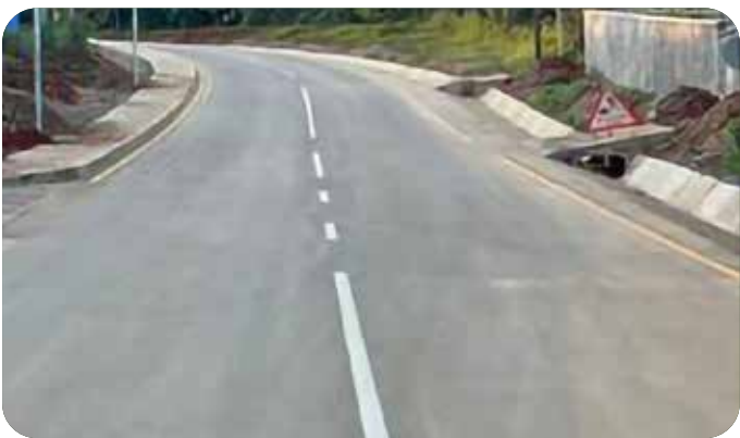
Figure 3: A completed section of asphalt surfacing, road markings and street lighting
