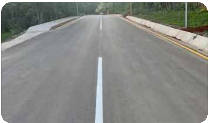
Figure 3: A completed section of asphalt surfacing, road markings and street lighting
