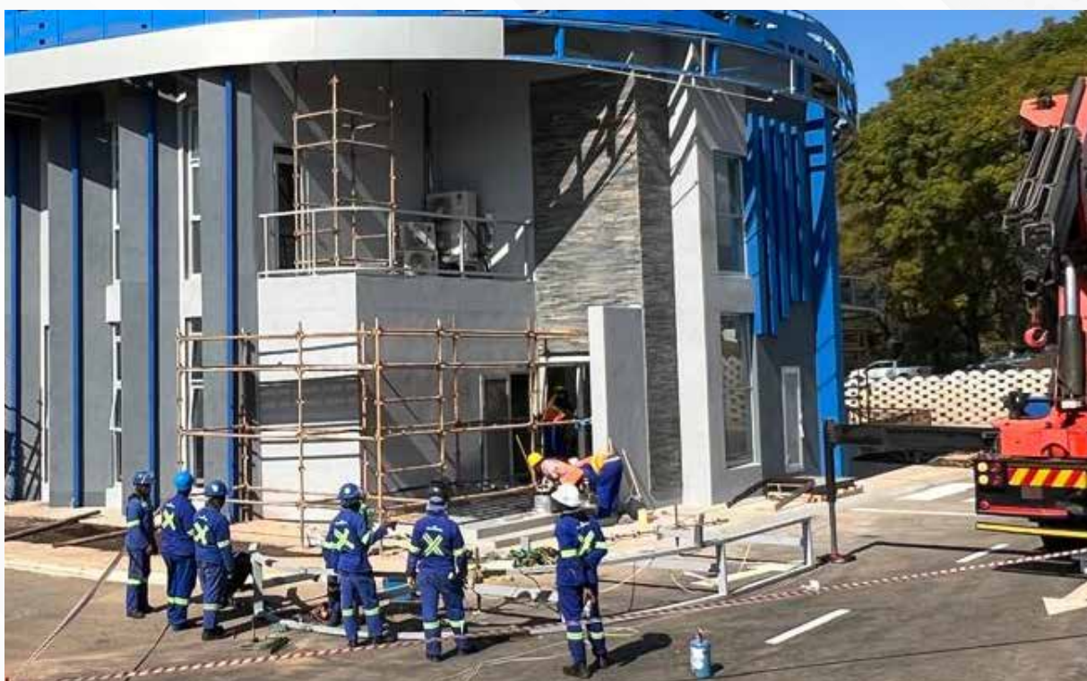
Figure 4 The development of Eswatini Water Service Corporation Office
