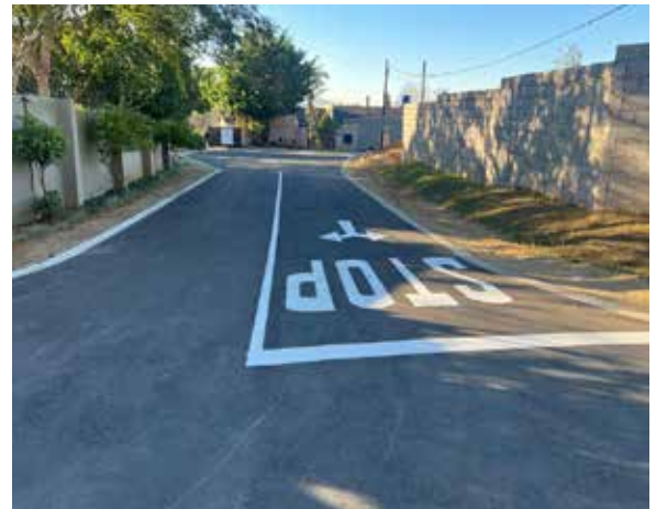
Figure 2: Rehabilitated Mantenga Drive and Mdzenga Close.
